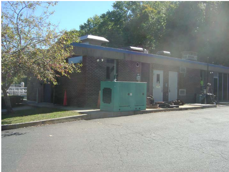
Photo 10: South Street WWTF Standby Generator next to Old Control Building
