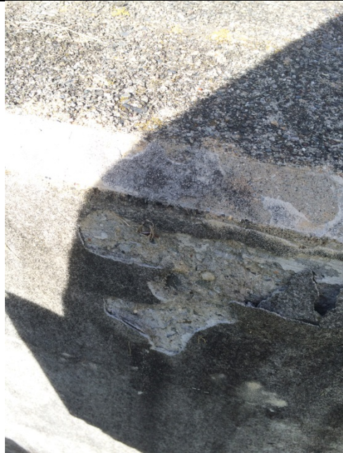
Photo 4: Route 7 WWTF – Primary Settling Tanks Concrete Delamination
