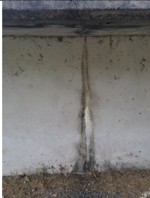
Photo 8: Route 7 WWTF - Equalization Tank Cantilever and Wall Concrete Cracking
