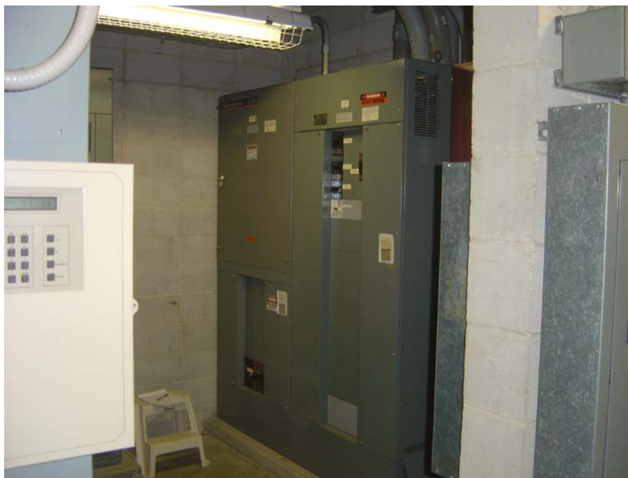
Photo 8: South Street WWTF Main MDP Located in Operation Building Electrical Room
