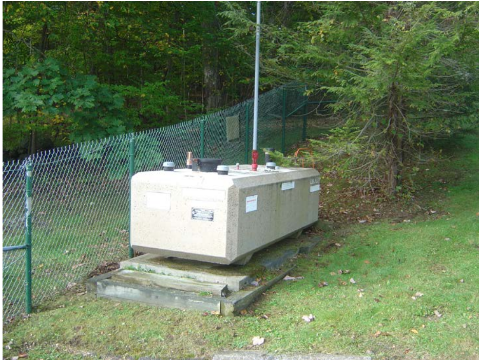
Photo 5: Route 7 WWTF Diesel Storage Tank
