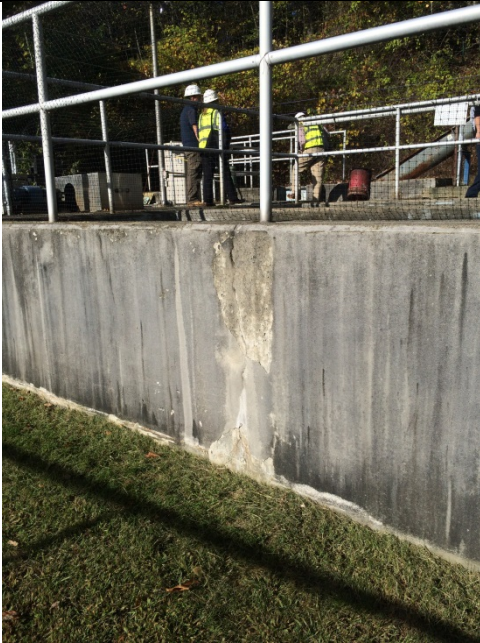
Photo 3: Route 7 WWTF – Primary Settling Tanks Delamination
