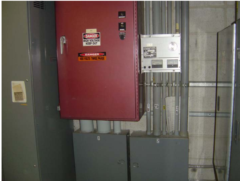
Photo 9: South Street WWTF ATS Located in Operations Building
