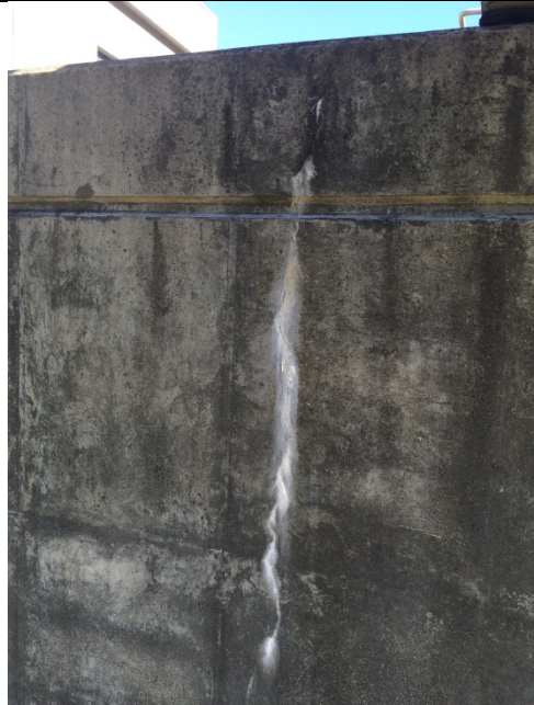
Photo 12: South Street WWTF - Aeration Tank Cracking
