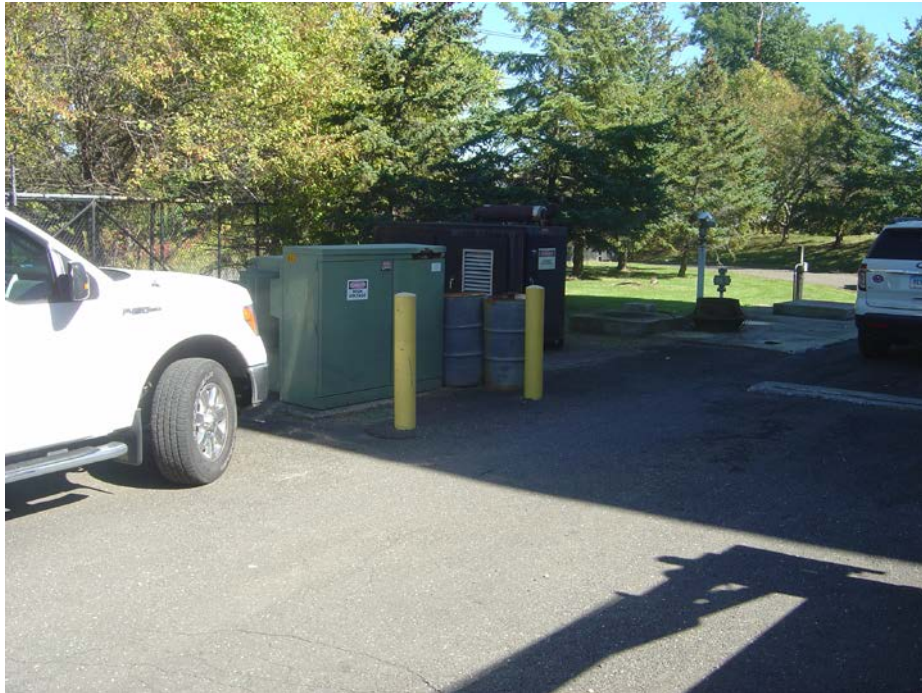
Photo 7: South Street WWTF Main Utility Transformer and Standby Generator Located next to Operations Building
