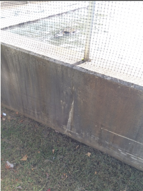
Photo 5: Route 7 WWTF - Equalization Tank Concrete Cracking
