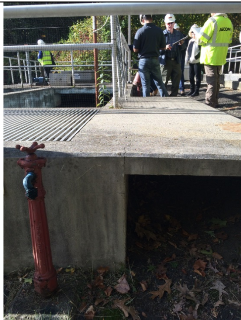
Photo 2: Route 7 WWTF – Primary Settling Tanks Cantilever Slab
