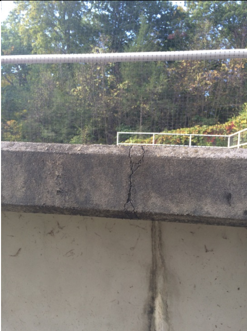
Photo 7: Route 7 WWTF - Equalization Tank Cantilever and Wall Concrete Cracking
