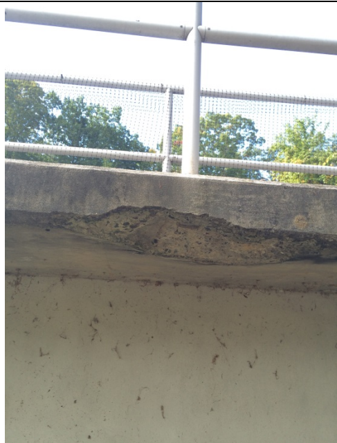
Photo 6: Route 7 WWTF - Equalization Tank Cantilever Slab Concrete Blowout
