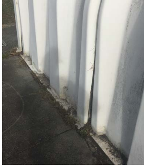
Photo 2: Route 7 - Rotating Biological Contactors cover seam
