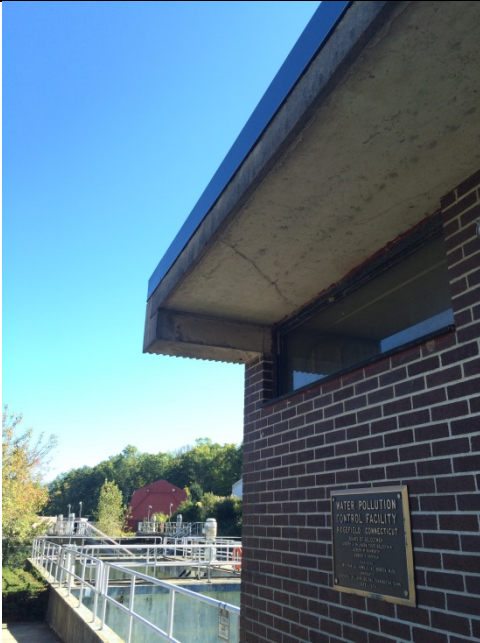
Photo 11: South Street WWTF - Control Building Roof Plank Crack
