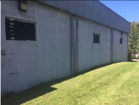
Photo 13: South Street - Operations Building EIFS damage
