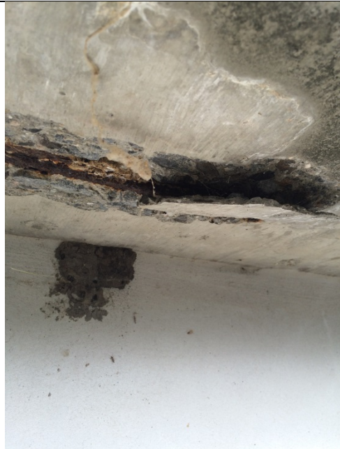
Photo 10: Route 7 WWTF - RBC Tank Cantilever Slab Delamination
