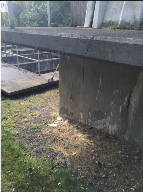
Photo 9: Route 7 WWTF - RBC Tank Cracking and Delamination
