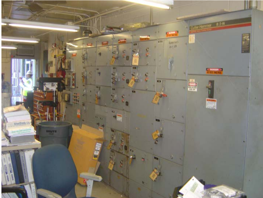
Photo 13: South Street WWTF Old Control Building MCC
