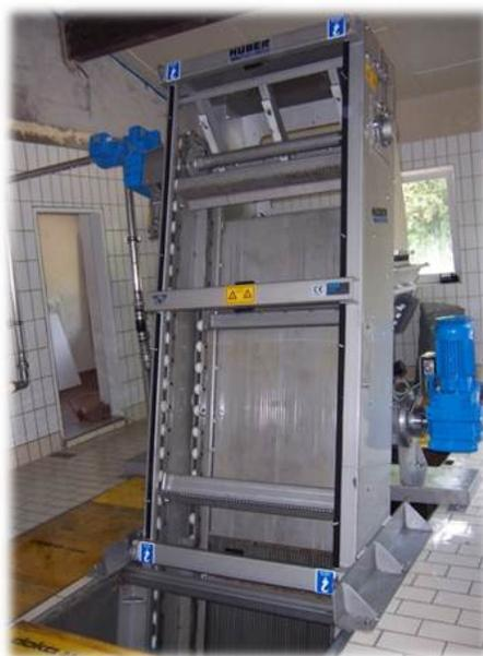
**FIGURE 6-2. MECHANICALLY CLEANED BAR SCREEN**
