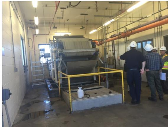
**FIGURE 5-11. SOUTH STREET WWTF SLUDGE BELT THICKENER /PRESS**
