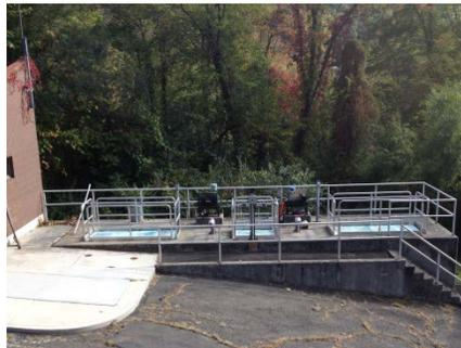
**FIGURE 5-5. ROUTE 7 WWTF SLUDGE STORAGE TANKS**
