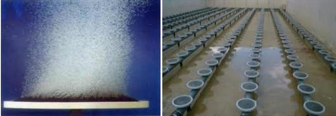
**FIGURE 7-20. FINE BUBBLE AIR - MEMBRANE DIFFUSER AND MEMBRANE GRID INSTALLATION**
